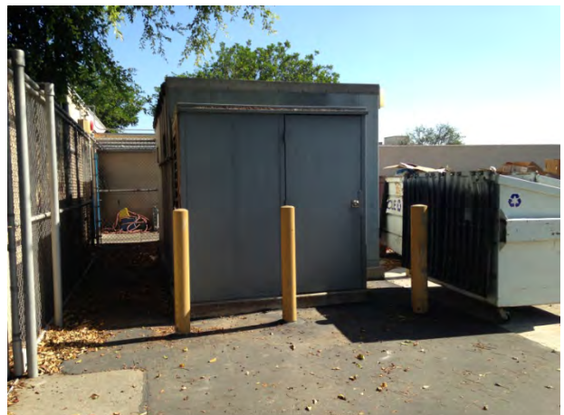
Figure C8: Refrigerator south of kitchen, facing east.
