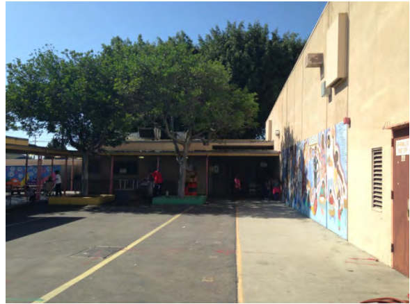
Figure C4: South of Auditorium, facing west toward Kitchen.
