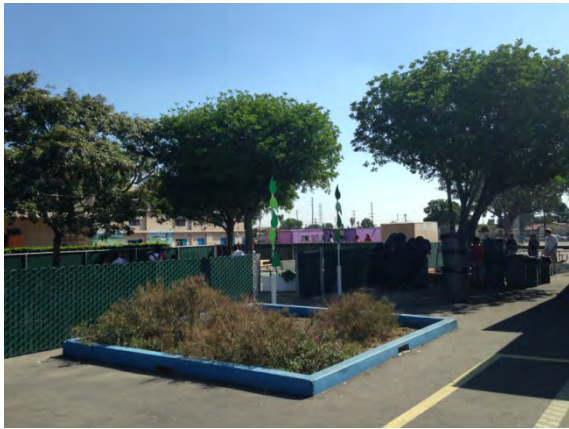
Figure C3: South of Auditorium, facing Southeast toward playground
