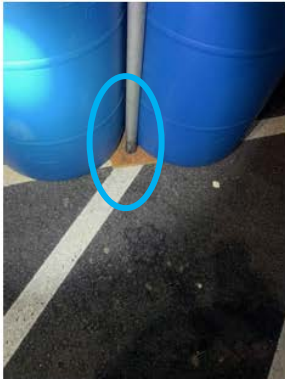
1. Tent pole in place on plywood plate as designed
