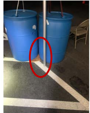
3. Tent pole knocked off plywood plate
