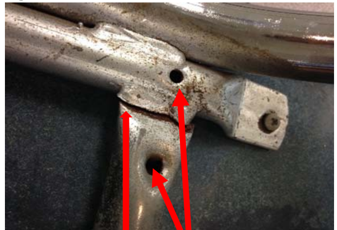
Broken weld Missing screws
